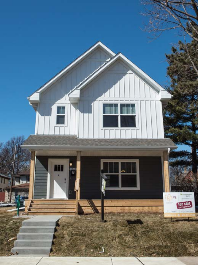
A new PRG construction in North Minneapolis.
